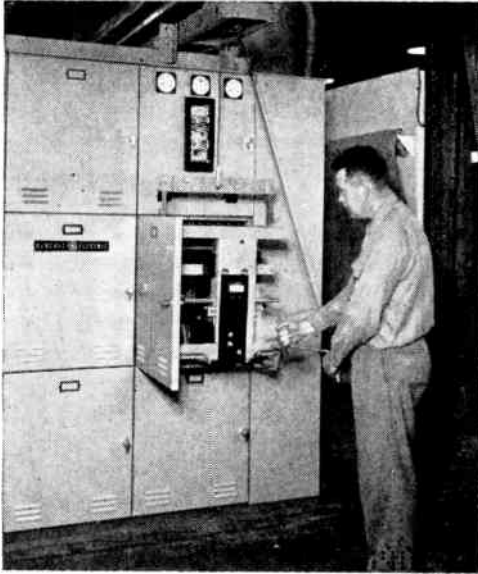
Installation view of a metal-enclosed, low-voltage, drawout air-circuit breaker switchboard.
