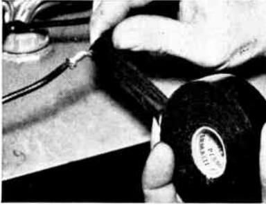
Permaccel 29 used as insulation in a wire splicing application.
