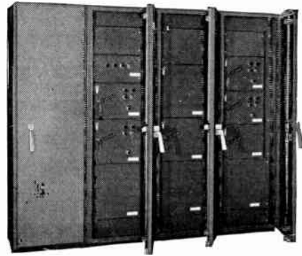
NEMA 5 Dust-Tight Control Center for Excessively Dusty Locations
