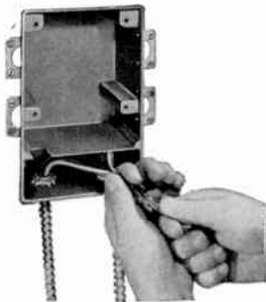
1. Attach wallbox to studs . . . feed input and output load BX through knockouts.
