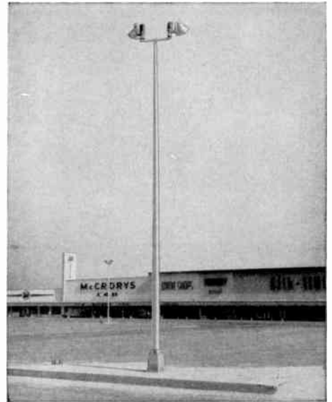
Aluminum Floodlighting Standards
