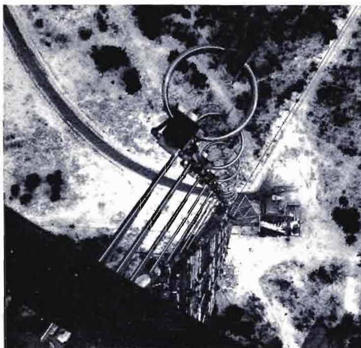
WGAN-FM, Portland, Maine—Gates 40 kW FM transmitter (above right), plus the Cycloid and vertical antenna combination (above left), 1460 ft. above average terrain, produces a 100,000 watt ERP signal.
