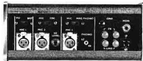
The rear panel shows the logical grouping of line terminations.
