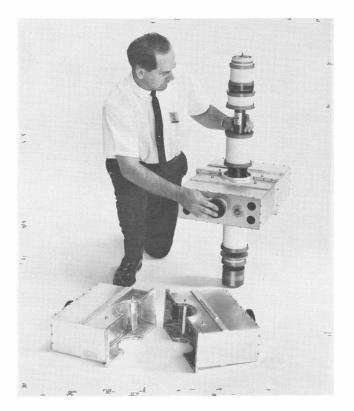
Figure 7—Typical Eimac Klystron and One of Its External Cavities Before and After Assembly.
