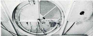
Above. Convenient access to antenna interior is through screened hatch. The eight point bearing check may be made without leaving the house by turning the outer shell with crank supplied.
