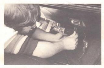
After fastening the mounting bracket to the dash with suitable bolts, mount the radio in the bracket and adjust it to a comfortable angle for viewing and operating.
