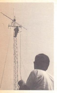
When working on any antenna tower a safety belt is a must.
