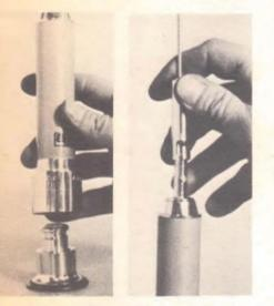
A low profile mount is a less obvious invitation to a would-be thief than a complete antenna waving in the breeze. Antenna Specialists' M-460 has a keyed arrangement to permit only the owner to remove it when parking. The M-450 is a quickrelease kit for instant whip removal.
