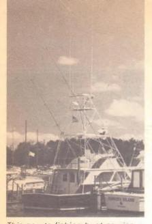
This sports fishing boat carries antennas for low frequency SSB, VHF/FM and CB communications plus radar.
