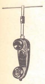
Stewart Warner Portafone was an early hand-held CB. The Portafone was also a Class B unit and sold for about \$200 a pair. Stewart Warner also made 6 and 12 VDC and 115 VAC power packs to operate the Portafone as a mobile or base station.
