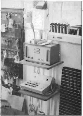
Hospital paging control. Lower unit selects individual bleeper by keying in required identity number. Upper unit sends all numbers for bleepers in cardiac arrest team. (Note tulip mike for transmitting location and type of emergency.) Spare bleepers for off duty staff are stored above being trickle charged.
