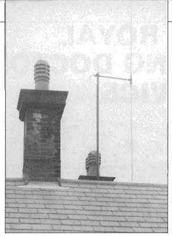
Antenna mounted on top of hospital complex (vertical dipole, centre fed).
