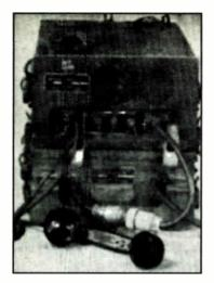
The famous BC-659 portable FM transceiver was typical of the mobile communications gear on 27 MHz used during WW II. It could operate up to 39 MHz.
