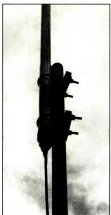
A look at the base of the completed assembly. The antenna mounts to a pole/mast using the provided hardware. (Photo by Harold Ort)
