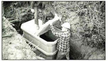
Hundreds of thousands of miles of fiber optic cable have been laid throughout the country with COMPOSOLITE® polymer concrete splice boxes placed about every two miles to house cable.
