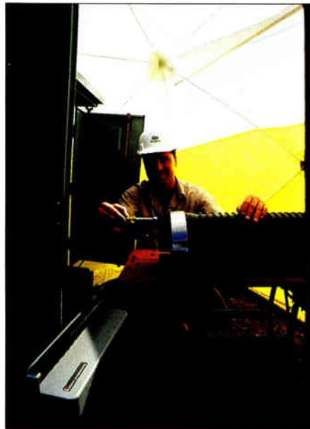
A technician prepares fiber for splicing.
