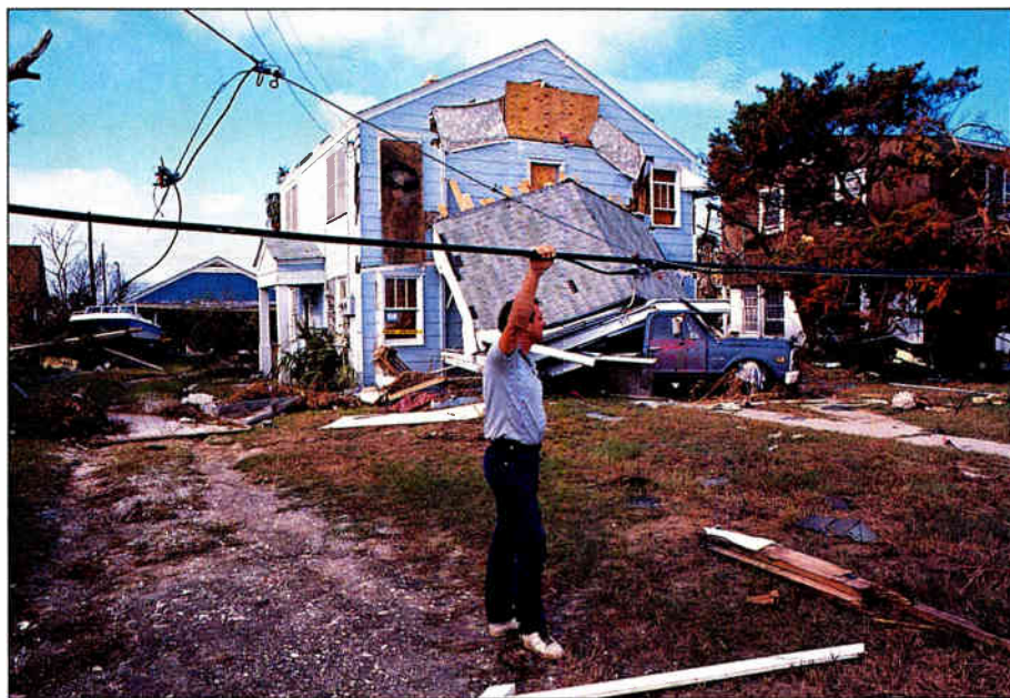
Charlie Jones, of Storer, evaluates damage caused by fallen trees
