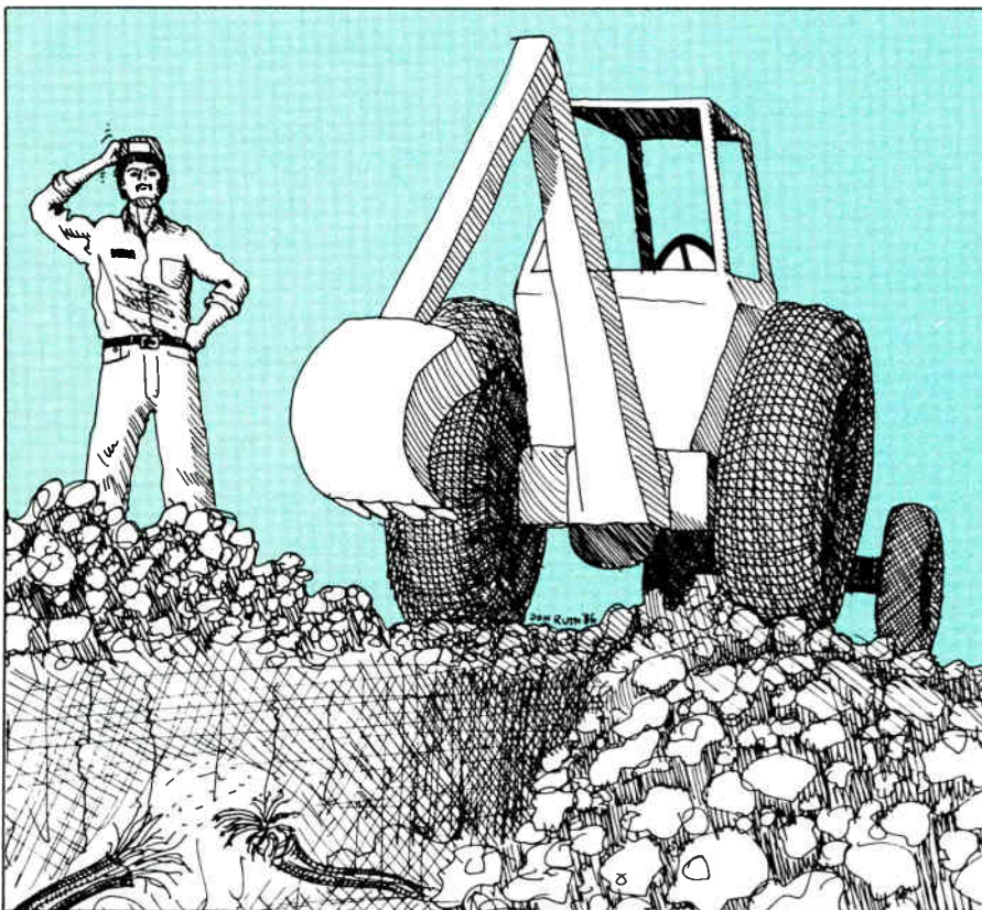
Trench digging often results in cable outages.
