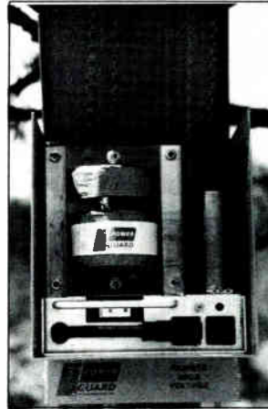
MODEL NS-6015-0 FERRORESONANT POWER SUPPLY
