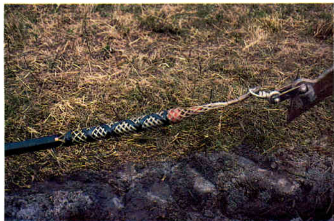
Coax-Cablecon can be plowed-in or laid in open trench if soil will not accept cable plow. Either way, continuous one-piece Coax-Cablecon beats hand work required with metal or PVC duct.
