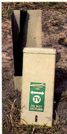
If trench depth exceeds minimum bend radius of Coax-Cablecon, no sweeps or elbows are needed for easy, continuous duct termination. Transition fittings are available for joining to other systems.
