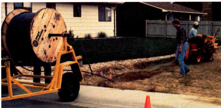
Coax-Cablecon makes for a fast installation: it arrives at your job site on reels, pre-cut to 1200 or 2400-foot lengths. Small back-lot tractors can plow-in Coax-Cablecon up to 60% faster than other in-duct buried systems: in-field demonstrations have averaged 60-feet per minute in medium density soils.
