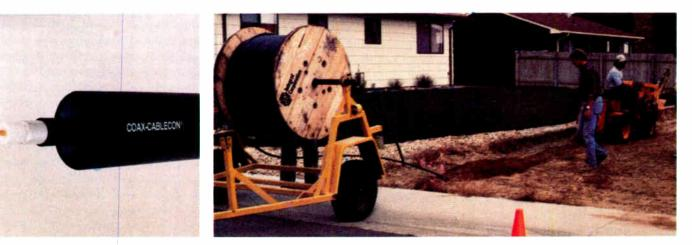
Coax-Cablecon duct is extruded over single, dual or multiple coax cable. Duct protects coax during shipment and in the ground. Coax-Cablecon makes for a fast installation: it arrives at your job site on reels, pre-cut to 1200 or 2400-foot lengths. Small back-lot tractors can plow-in Coax-Cablecon up to 60% faster than other in-duct buried systems: in-field demonstrations have averaged 60-feet per minute in medium density soils.
