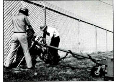
A.B. Chance Company anchor installer
