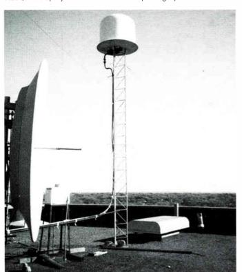
Radar antenna with dome
