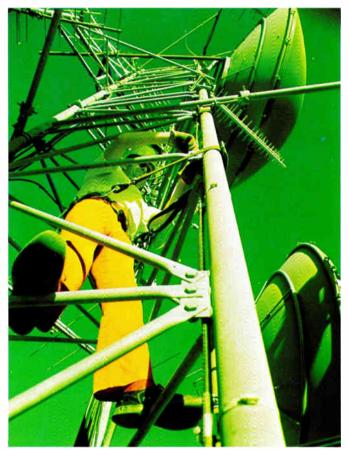
Technician aligns antenna to bring in path signals to receiver site.
