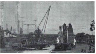
1:33 PM/OFF LOADING TVRO...Now the concrete is drying and the twin half-sections of the USTC SAT/FLECT I steel TVRO are off loaded from the lowboy trailer and placed into position adjacent to the poured base piers.
