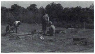
12:22 PM/READY FOR CONCRETE...Three concrete piers will be poured using 5.5 cubic yards of 3500 pound (2% calcium for quick-drying) concrete. 3,000 pounds of steel TVRO will sit here in six hours.
