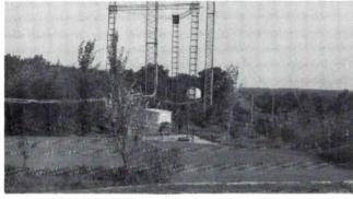
**10:59 AM/THE SITE...** Stakes in place, at 11 AM USTC will appear with a transit and locate the base center line. The terminal will go just behind the small tree left of center.
