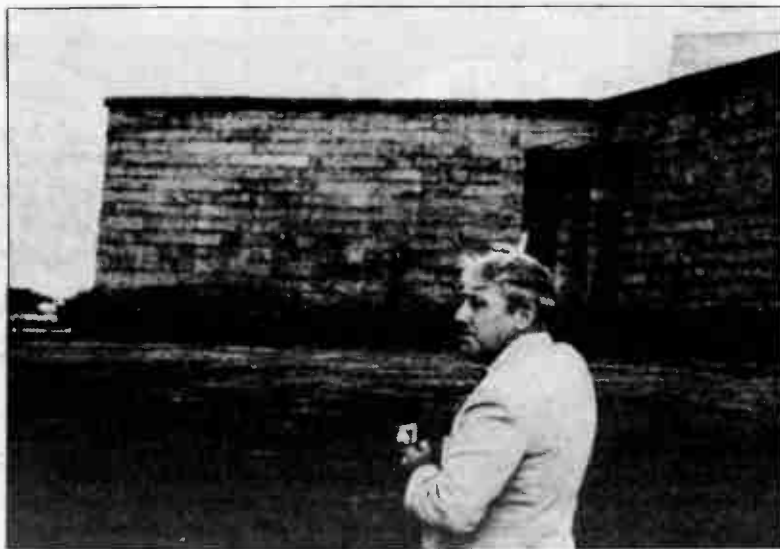
Kontoleon points out deterioration in the Statue of Liberty.
