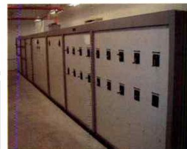
CUSTOM PHASOR INSTALLATION
