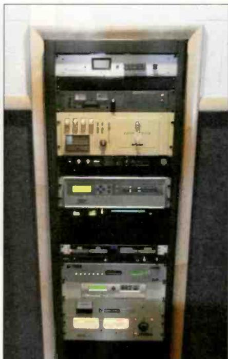
A single rack in the AM control room houses the STLs, some audio processing and other central operating equipment.
