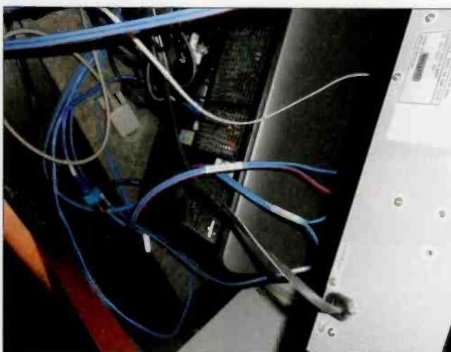
Wire labels make it easy to identify the function of any cable.
