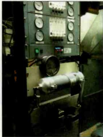
Unfortunately, the compressor units contained in the Andrew Dryline systems are made by a predecessor of Thomas Industries, which is in the process of moving and has allowed its parts inventories to dry up (no pun intended). Extensive searching proved these compressors to be rare and their parts even rarer. Rebuild kits from Andrew are priced somewhere north of \$1,500 and include nearly every active part of the system. I clearly needed another solution.
