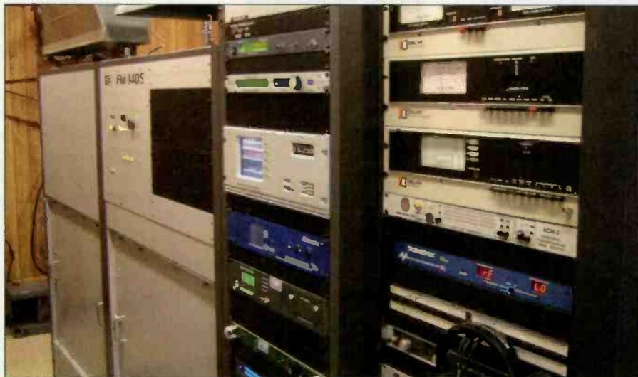
Broadcast Electronics FMI-1405 IBOC transmitter and associated equipment at repeater station WKSU
