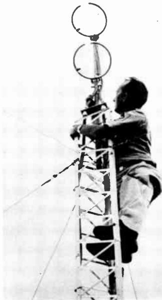
Fig. 2-15. Antenna Installation of United States Air Force TV Station, CSL-TV, Azores. The Rings are Separately Excited from Aural and Visual Transmitters. Official United States Air Force Photo.
