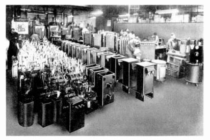
Fig. 11-17. Testing and tank (case) assembly room of a transformer manufacturer. (Courtesy of Eisler Engineering Company.)
