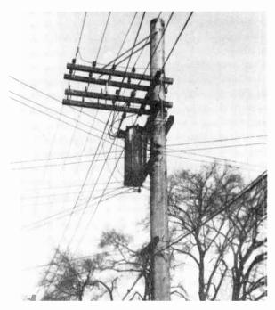
Fig. 11-39. A distribution tronsformer mounted on a pole.
