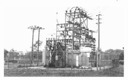
Fig. 11-40. A typical substation where several power transformers are used. (Courtesy of Kuhlman Electric Company.)
