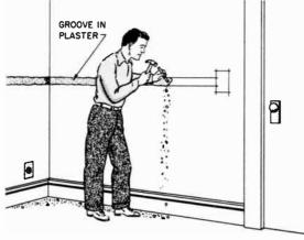
Fig. 15-38. Grooving plaster to make an electrical extension.
