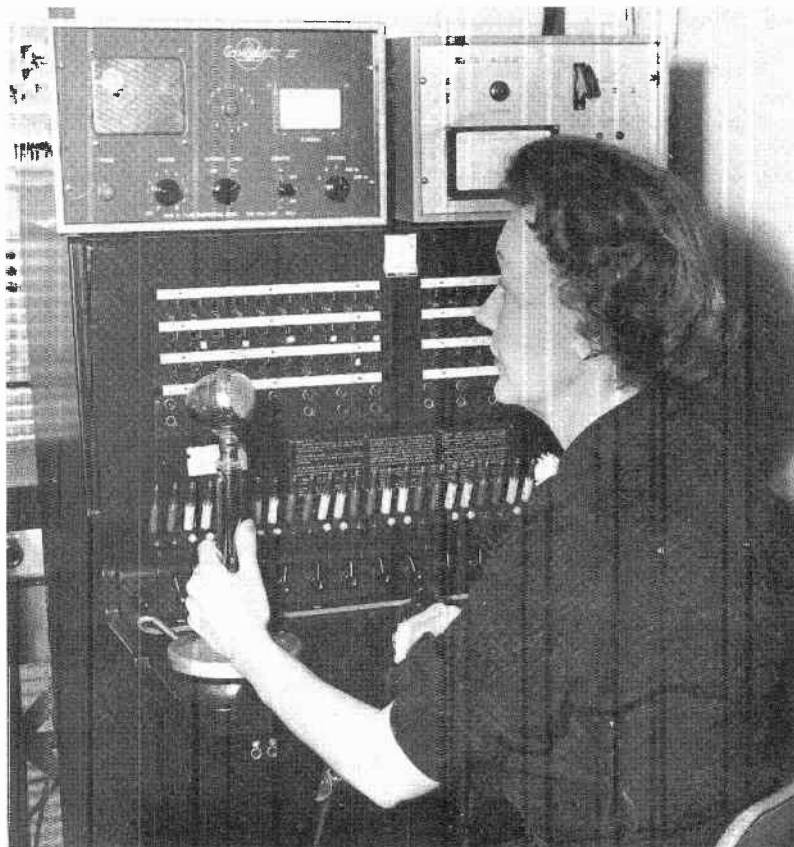
Fig. 1-11. Radio paging system in a telephone answering service. (Courtesy of Kaar Engineering Corporation.)
