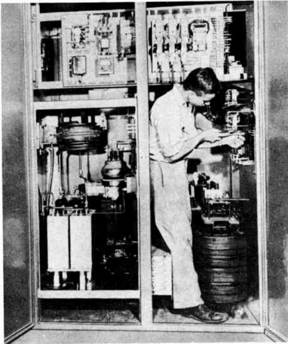
Fig. 103. Large induction generator being adjusted by technician. (General Electric Co.)
