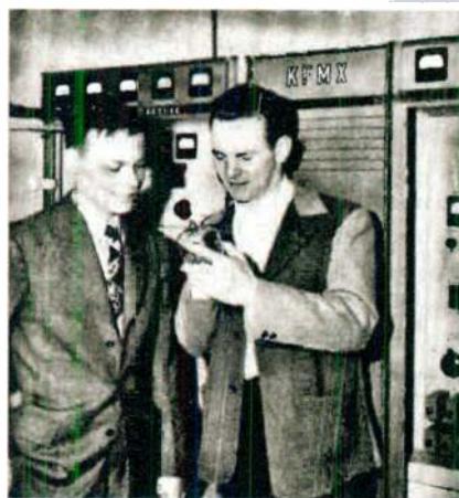
Engineers at the KFMX transmitter, co-located with KSWI 1560 transmitter on the South Omaha Bridge Road, 1948.
