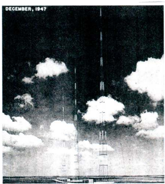
1947: KFAB's three-tower transmitter site on the south edge of Omaha in Sarpy County.
