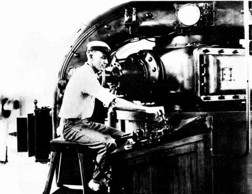
Pl. 7: At the controls: Operating a 500 kilowatt Federal arc.
