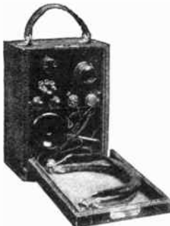
Model P-11 One Tube Portable—the Camera of Radio. Price, $16.00 without accessories. Tube, batteries, head phones, antenna, and ground wire all self-contained. Weight 4½ lbs. complete.
