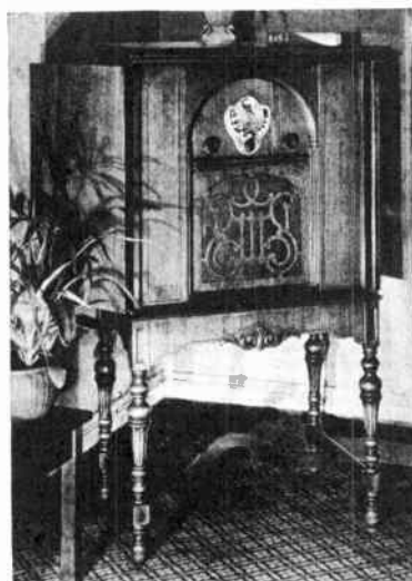
K-43 —Handsome cabinet with doors of figured butt walnut and two tone panels. Seven tubes and rectifier. Selector tuner. Dynamic reproducer. Screen grid tubes. Push-pull amplification with 2 type 345 tubes. $235 00 Price, less tubes . . . . .
