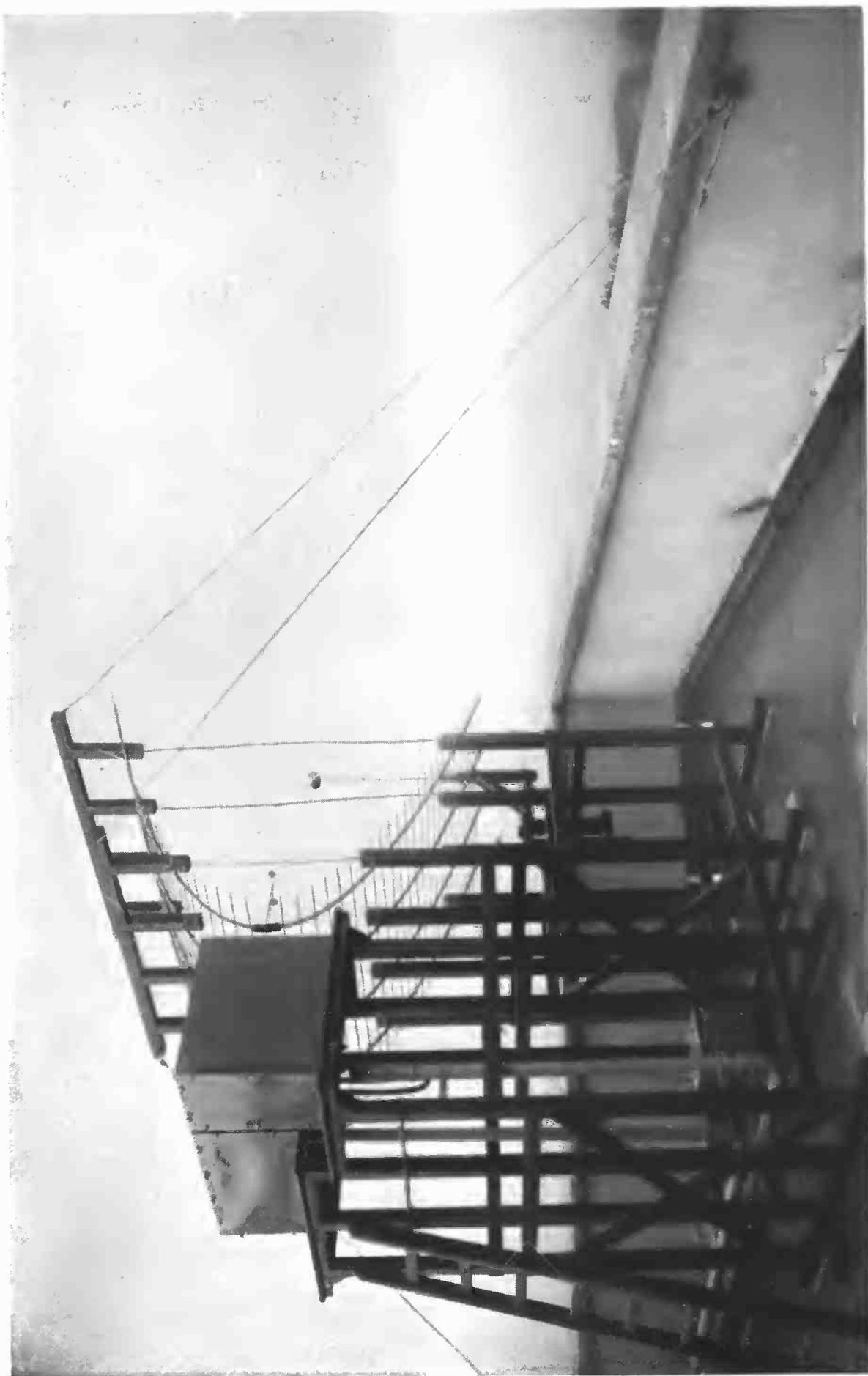
Marconi ultra-short wave reflector or radio "searchlight" on top of the Vatican station "beams" a 56-centimeter wave across a distance of about fifteen miles.
