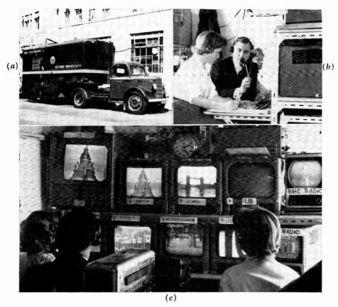
Fig. 20-35. Main BBC control center for the royal wedding. (a) Outside Broadcasts van outside Broadcasting House. (b) Peter Dimmock, head of Outside Broadcasts, at control desk with two assistants. (c) Mr. Dimmock faces an array of 10 monitors displaying the various inputs and outputs to the switching center. Pickup from the Tower Bridge (top center monitor) does not show on the chart. The purpose of this was to show the royal yacht leaving for the honeymoon.
