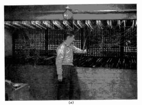
Fig. 18-16. (a) An NBC patchboard. This board provides for the patching of 1,200 individual lamp circuits. Plugs above and below are connected to individual lamp outlets. Receptacles at back are connected to source of power through dimmers and switches. (b) An NBC dimmer board comprising 36 individual autotransformer dimmers plus master and submaster controls.
