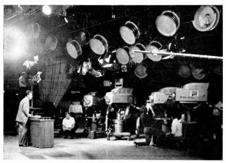
Fig. 21-1. At least four times as much light is needed for NTSC color TV, necessitating the use of many 5,000-watt floods and spots and much flat lighting. The large floods are not lighted above because of the small playing area. Two senior (5-kilowatt) spots, one from each side, give essentially flat front light. Modeling is achieved by other seniors used as kicker and back light (this is revealed by the shadows of the desk). (Photo courtesy of NBC.)
