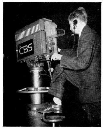
Fig. 4-11. Pat McBride adjusts pedestal height while his camera is on the air. (Courtesy of Popular Science.)
