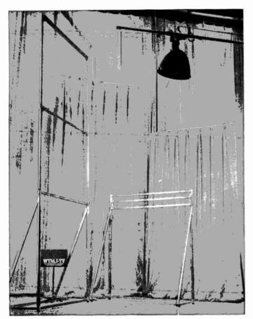
Fig. 16-11. Magnesium frame screens at WTMJ-TV, Milwaukee. Photo shows same type of screen draped and undraped and at different heights.
