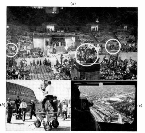
Fig. 20-38. (a) Interior of sports arena at start of session. Circled are the three major camera positions surrounding podium (arrow). At top of picture large screen TV projection can be seen. (b) Mobile camera outside sports arena mounted on Fisher mike-boom base. (c) CBS cameraman in blimp picks up aerial view of Los Angeles sports arena during 1960 Democratic convention.
