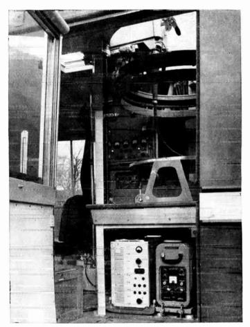
Fig. 20-17. Interior of BBC Roving Eye. Camera well and part of camera, which protrudes through roof, can be seen. Camera is roller-mounted on a circular track, so it may be swung around to face any direction, while the operator remains always behind it. Vertical adjustment screw shows at left of track.
