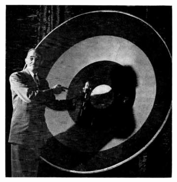
Fig. 19-5. Microphone placed at focal point of parabolic reflector for highly directional pickup.
