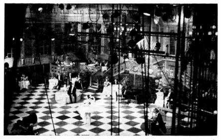
Fig. 18-11. Lights mounted on counterweighted battens (ABC-TV, New York, Studio 1).
