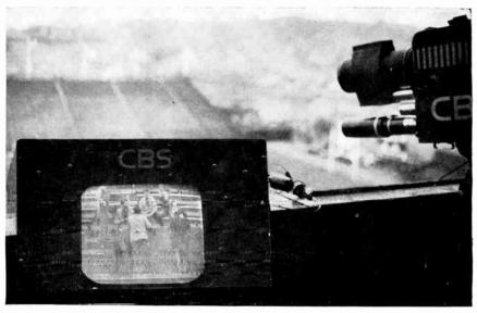
Fig. 5-5. Video Reflectar lens (early model) focused on people in the stands across a football field. The camera's picture is visible on the monitor in the foreground.
