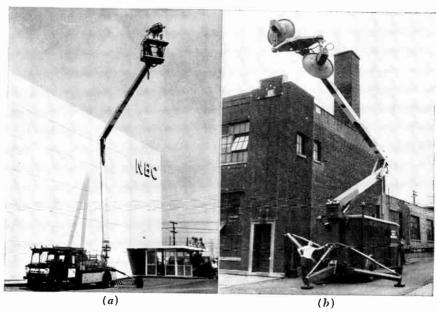
Fig. 20-23. Extra height. (a) NBC camera rises 75 feet on high-reach apparatus from Sign Maintenance Company. (b) Similar equipment used by Illinois Bell Telephone Co. to raise microwave transmitters to the same height.
