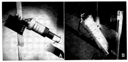
Fig. 18-25. Fuddle projectors, using PAR 38 lamps. (A) Fastened to standard clipon shield and supported at the lamp socket; (B) heavier model supported centrally.
