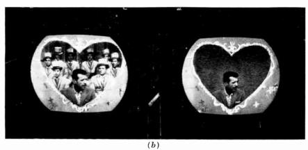
Fig. 15-11. Montage effect done in Chroma-Key on the "Tennessee Ernie Ford Show." (a) One camera shoots Ernie behind a heart-shaped gobo, the other frames the chorus. Monitor on left (b) shows composite result.
