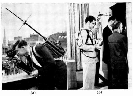
Fig. 20-4. Wireless TV cameras. (a) French radio-camera used by the BBC; (b) small experimental vidicon by RCA. Small electronic view finder is hung on chest.
