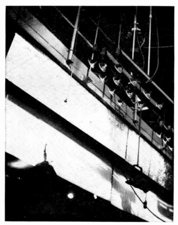
Fig. 18–5. Aluminum-foil reflectors used by Karl Weger of WPTZ. These were inspired by a stage-lighting technique used by Mariano Fortuny shortly after 1900, and have been nicknamed "Fortuny reflectors." The white board hanging below the reflectors is only a baffle to keep unwanted light off the studio beyond.
