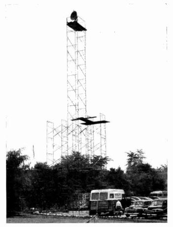
Fig. 20-22. Seventy-foot tower of scaffolding erected by WXYZ-TV, Detroit.
