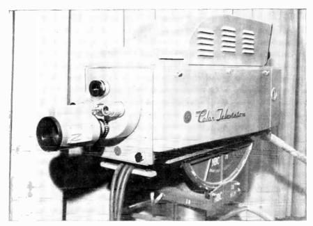
Fig. 5-11. Super Studio Zoomar lens on RCA color camera. Turret may be rotated for other lenses.
