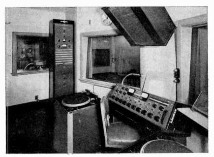
Fig. 14. Control console and rack, Station WUOM (Collins Radio). This control room serves two studios. WUOM has no master control. (University of Michigan.)
