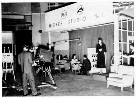
Fig. 24. Intra-store (closed-circuit) television. Dramatized commercial originating in the Highee Company School Salon. The program was speeded considerably by having the camera switch from the salesman starting to fit the shoes on the model to the second girl at the right wearing the shoes being described. (R.C.A.)
