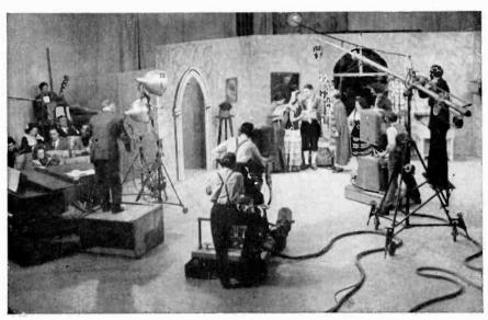
Fig. 38. This photograph in the studio of WRGB shows how compactly the actors are grouped. To the left is the orchestra for musical interludes and background. In the immediate foreground is a camera on a dolly; another camera is to the right; and the microphone boom to the extreme right is hung above the actors. (General Electric-WRGB.)
