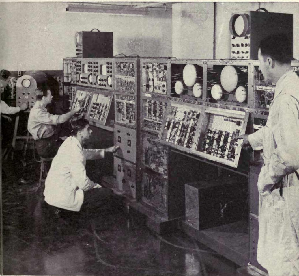
*The control room is a busy place, but no one rushes about. Each control operator must watch the screens to which he is assigned, and instantly select the scene which is best suited to be broadcast. A flick of a switch changes the broadcast from one screen to another.*
