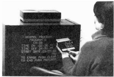
RCA introduces a remote programmable VCR with the Convertible VKP900. The unit uses a microcomputer chip that allows user to set the clock remotely and pre-program up to eight programs a full year in advance. Alphanumeric graphics appear on the tv screen, simplifying the programming process.
