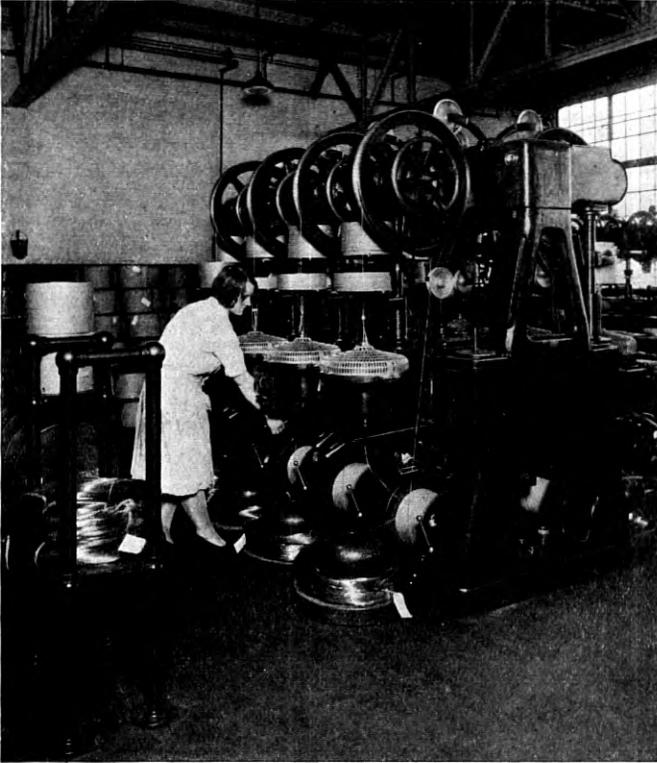
Fig. 6—Paper insulating machine.
