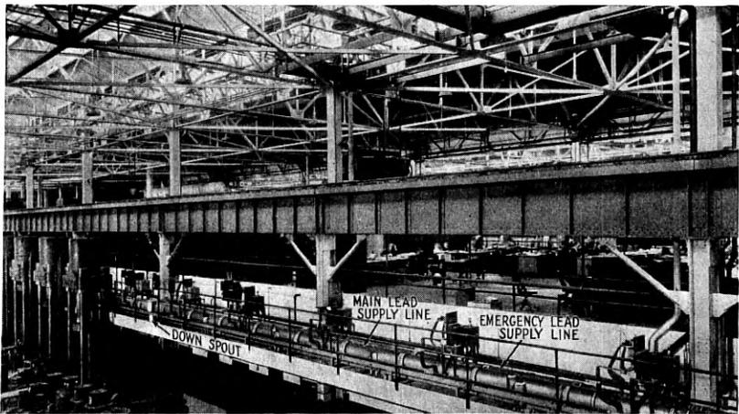
Fig. 28—Main lead supply lines.
