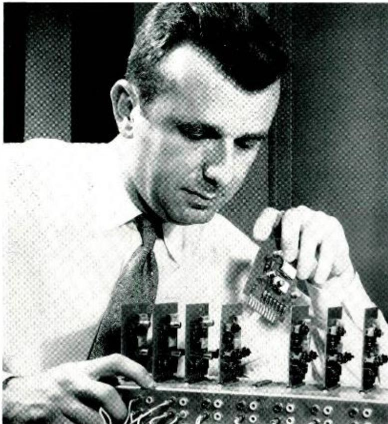
*L. D. Harmon assembling a network of electronic "nerve" cells. Such transistorized circuits simulate some functions of actual nerves.*
