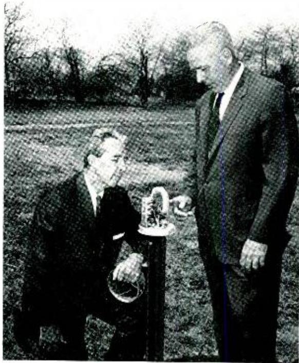
*C. C. Lawson, left, and W. J. Lally examining a post-mounted pedestal terminal. At these points service wires are connected to selected cable pairs.*
