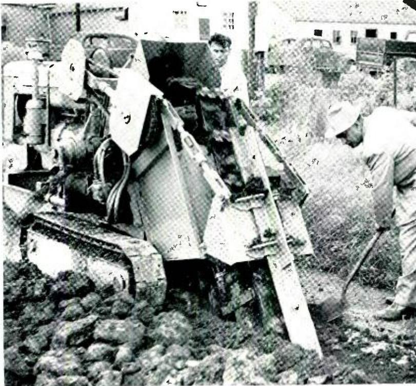
*A crawler-mounted trencher being demonstrated by the manufacturer. Different types of trenching machines are continuously studied as part of the program designed to discover the best-performing equipment for burying cables.*
