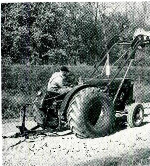
*Plowing of rural distribution wire in the Illinois countryside. A special plow, used here, has modified industrial tractor and special reel equipment.*
