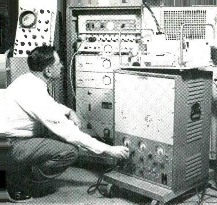
*Fig. 4 — The pulse receiver. E. J. Henley adjusts the attenuator in the power supply unit, on which is resting one of the converter-preamplifier assemblies. The oscilloscope at the far left stands beside an intermediate frequency amplifier and power supply unit.*
