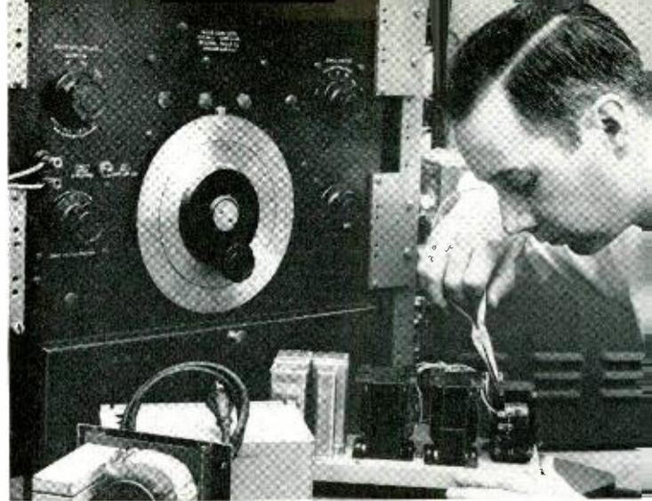
*Fig. 3 — W. T. McMahon changing connections on tone generator in preparation for measuring harmonic output.*
