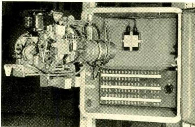
Fig. 2—Flat-gain regulator for the type-K carrier system
