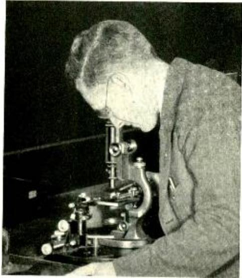
*R. M. Sample uses the micro-manipulator.* The crystalline structure of metals and metallic alloys is studied in minute detail; conclusions are drawn as to the causes for defects in metals; changes are seen due to various treatments of the metals; and improvements are suggested.
