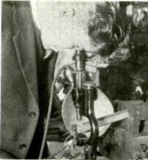
*A rubber-line recorder being adjusted by Harry Summers*
