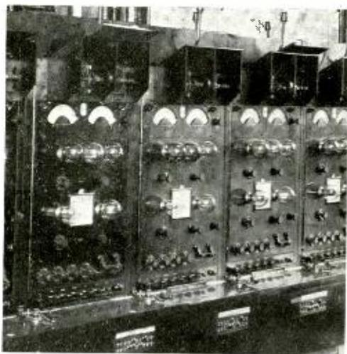
*Part of the Type A carrier telegraph terminal equipment at Pittsburgh*
