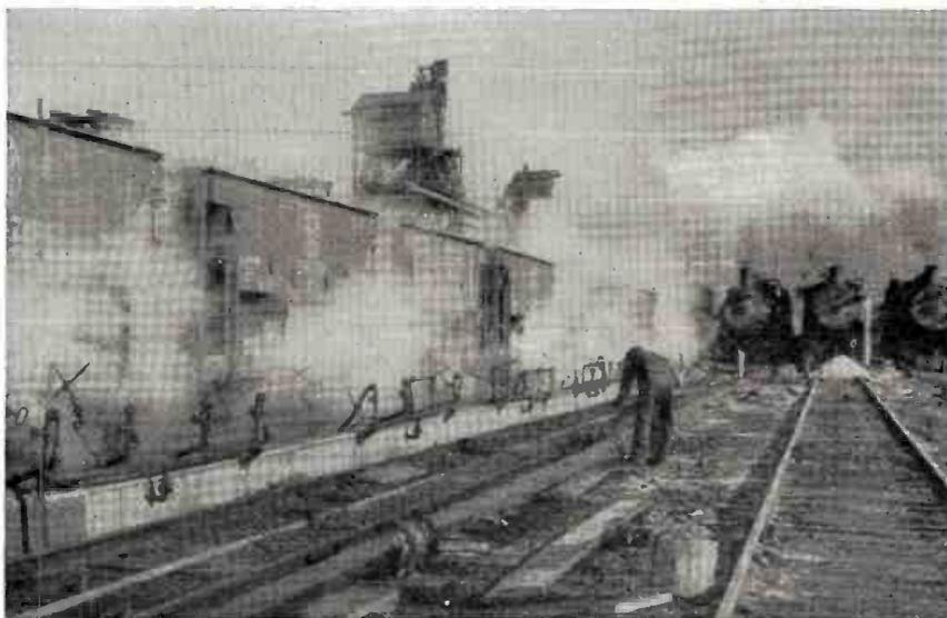
**2 MAKING HISTORY WITH STEAM:** New steel mills (and production from present mills) are going up so fast that the summer season of ore boat transportation needs to be stretched. This picture shows first winter-time trainload of frozen ore being given a steam bath for fast dumping.
