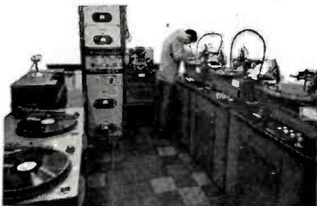
**The recording room at Indiana U., showing PRESTO disc recorders and reproducers, PRESTO rack mounted amplifiers and the famous PRESTO PT-900 portable tape recorder.**
