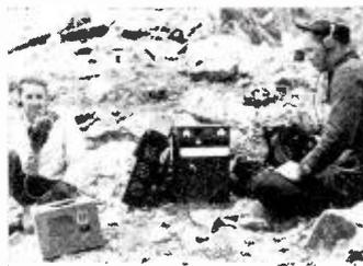
HIGH IN THE ROCKIES, in fact 13,000 feet high, was the origination point for a program during the annual trek of the Boulder (Col.) Chamber of Commerce. KOA, Denver, got its outfit up to this point on the Continental Divide by pack-horse. A relay point was set up 2½ miles below, with the regular lines another five miles down the mountain. Here Don Martin (left) and Engineer Verne Andrews operate the equipment.
