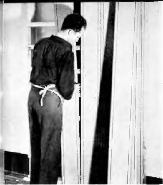
Bagasse (cane fibre) boards are easy to install and serve a number of important functions
