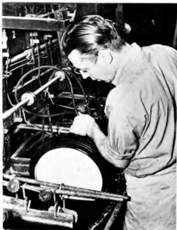
After the process of first copper plating the wax, having been treated for fourteen hours, is removed from the copper plating tank
