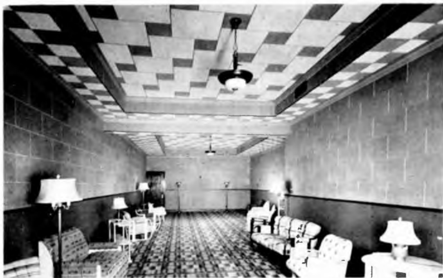
Acoustical material of the type shown here may be used throughout the store, or just in demonstration rooms or listening booths
