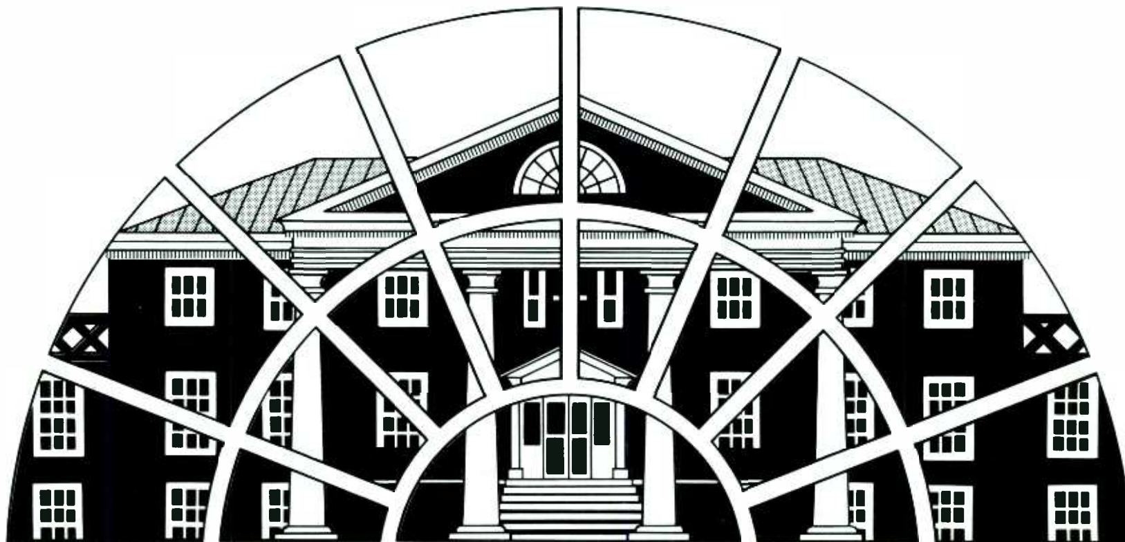
MONTPELIER, MONTPELIER STATION, VA.
