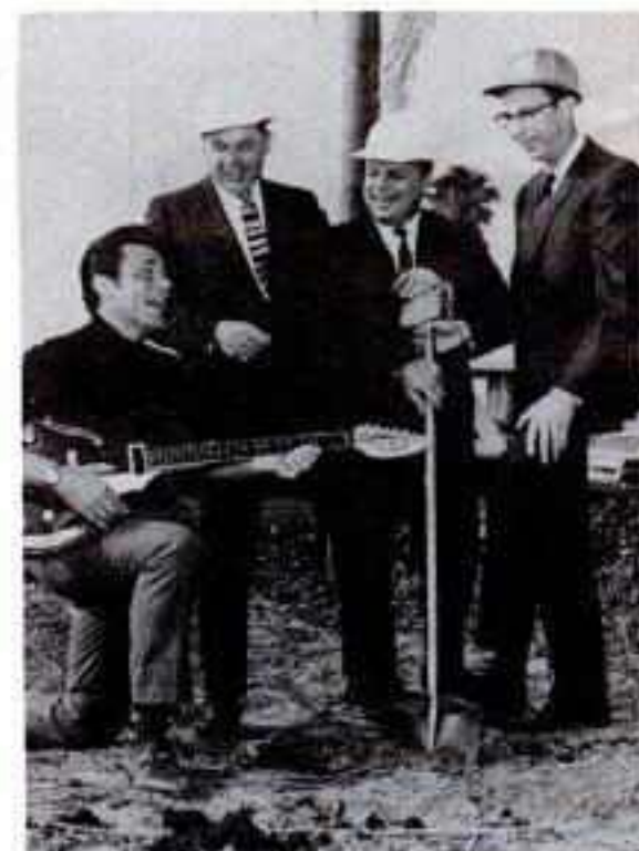
GROWTH OF THE THOMAS ORGAN CO. has resulted in the ground-breaking for a 9,000 square-foot, $152,000 addition to present Sepulveda, Calif., facility. Bill Page, kneeling, serenades, from left, Robert Bloomberg, president; David Heister, director of industrial relations, and Stanley Cutler, vice-president and director of design engineering.
