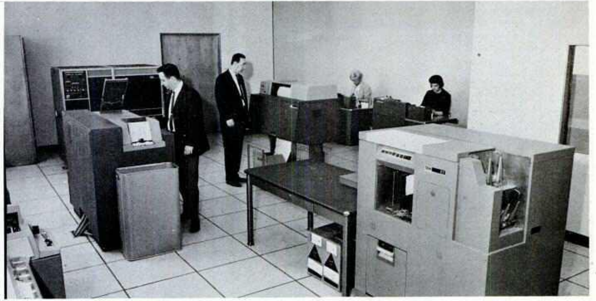
THIS $250,000 IBM ROOM has just been opened at the giant Rock-Ola Mfg. Corp. plant in Chicago as part of a two-year-old property rehabilitation program. This Electronic Data Processing Center, new offices for the production control department and the accounting department were in the latest phase completed in the program. Pictured in the environment-controlled EDP Center are, from left, an IBM 083 Sorter, an IBM 1402 Card Reader and Punch, an IBM Processor, an IBM 1403 Printer, the IBM 087 Collator and IBM 024 Key Punches and IBM 056 Verifier. Plans call for the installation of the IBM 360-20 memory disk unit.
