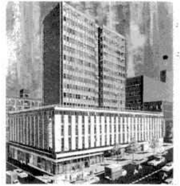
GALLO (AFRICA) LTD. moved into its new Johannesburg, South Africa, building on Oct. 3. The modern quarters include first-floor recording studios, which were designed by the firm's Council for Scientific and Industrial Research, which has a specialist acoustical department. The official opening of the new structure is set for Dec. 20.
