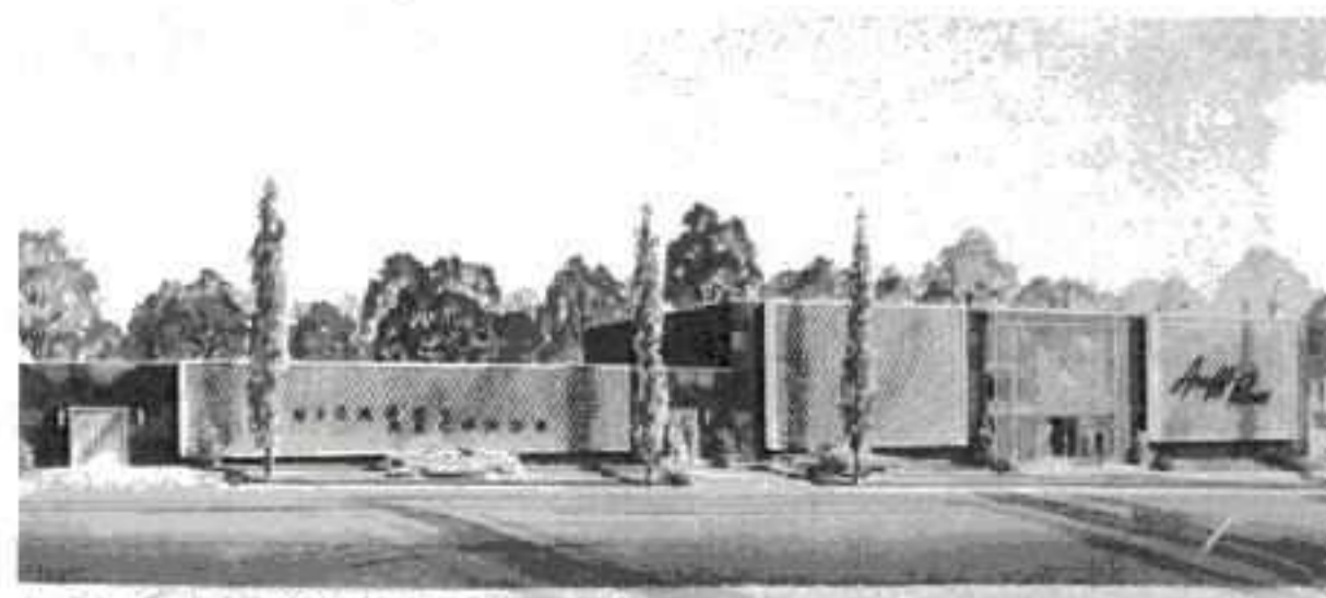
GROUNDBREAKING CEREMONIES are scheduled Wednesday morning (19) for a new $400,000 building for Acuff-Rose Publications, Acuff-Rose Artists Corp., and Hickory Records. Building is to be ready by May, 1967. It contains 40 offices, conference rooms, studio, and mastering facilities. Roy Acuff and the Smokey Mountain Boys will entertain at the ceremonies.
