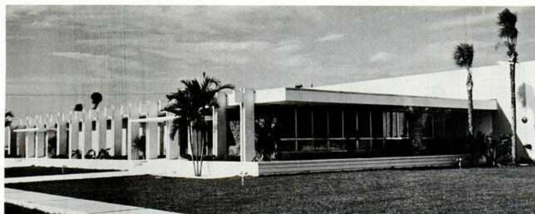
NEW MIAMI headquarters of Mar-Tab is set in the Sunshine Industrial Park.
