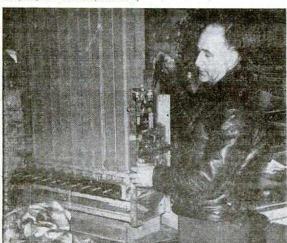
CANDY MACHINES OPERATED by Aaron Strouse are regularly pulled in to his shop for servicing and routine maintenance. Here Strouse adjusts the coin mechanism on an overhauled multicolumn vender.
